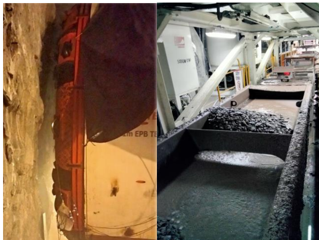
Figure8. Excavation, Muck Transporting & Disposing
