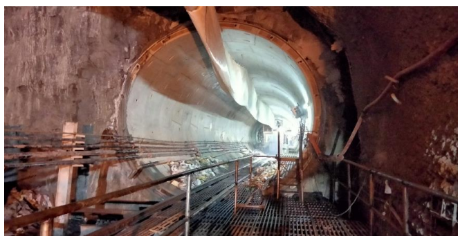
Figure 9. Downline Tunnel at Swarget Station
