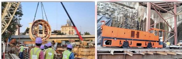
Figure 4. Lowering of TBM & Locomotive
