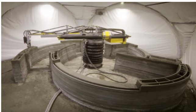
Figure 20 During 3D printing process
