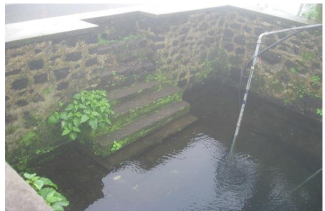
Rock-cut water cistern with dressed stone walls at Sinhgad fort. (Source: India Water Portal)
